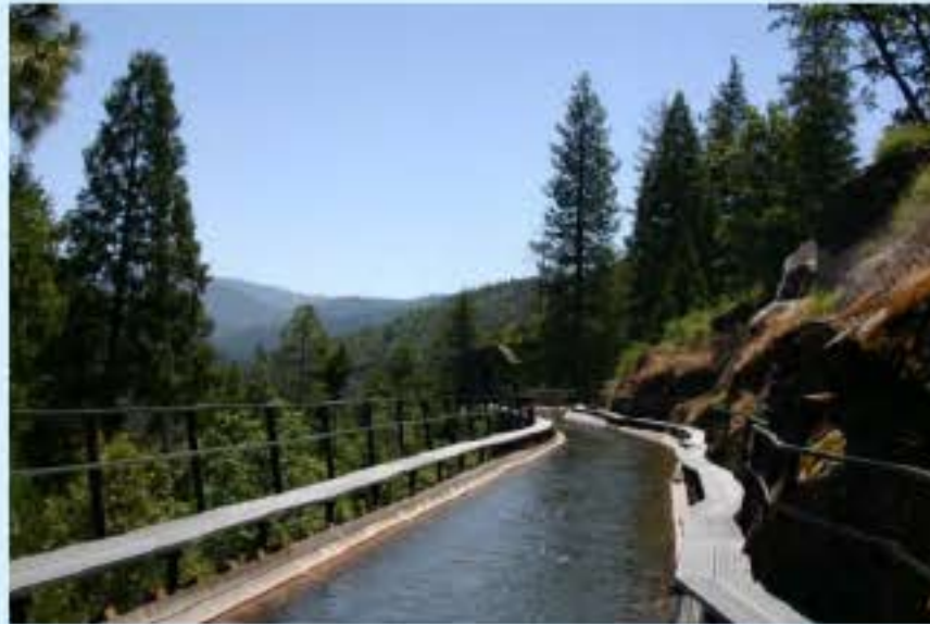
A flume carries water from the high country to reservoirs and treatment plants
